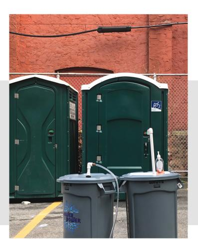
To respond to the widespread closures of public restrooms, we worked with LavaMaeX to design and build four hand-washing stations, operated with a foot pump.
